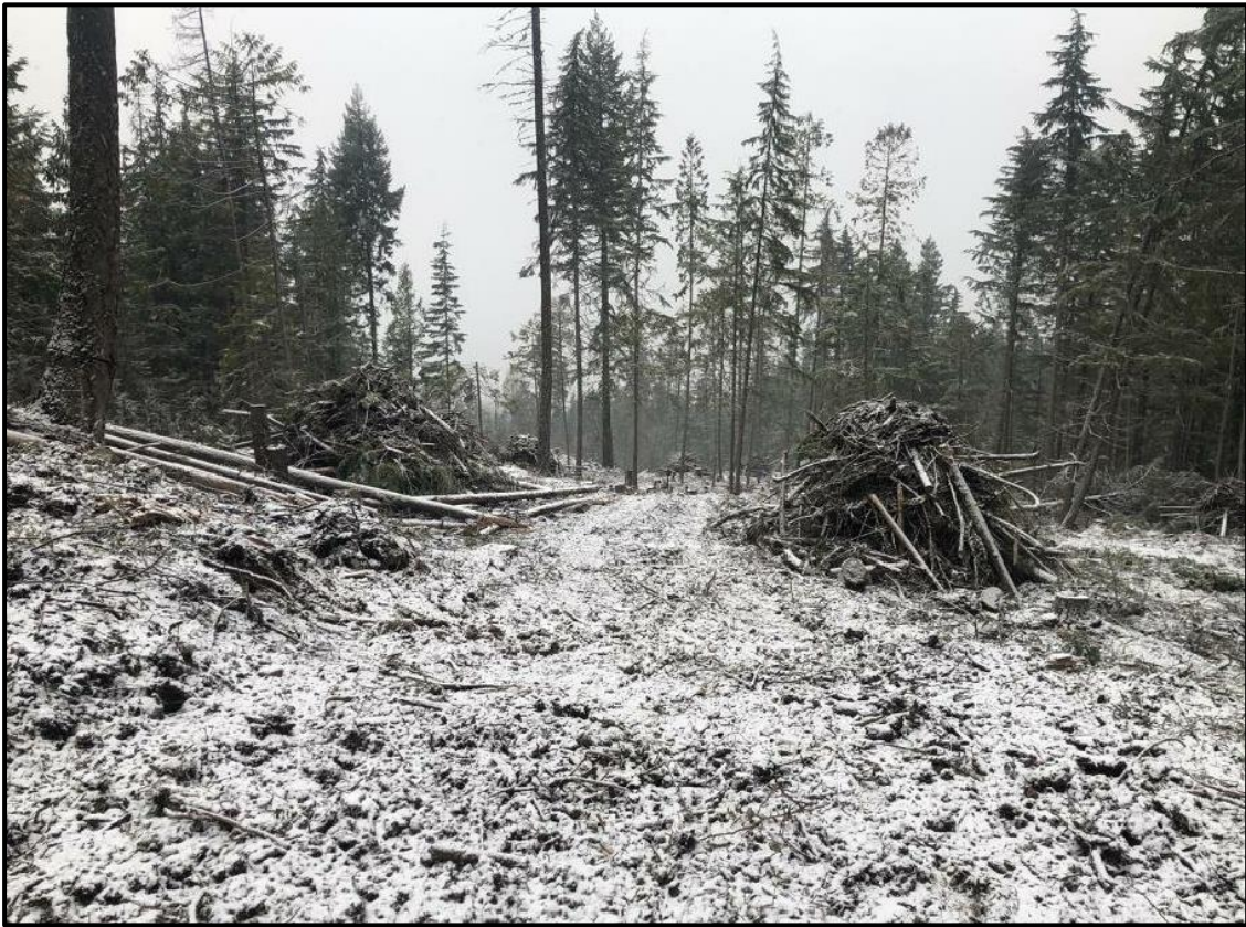
Debris piling completed, trail left in place for wildfire access
